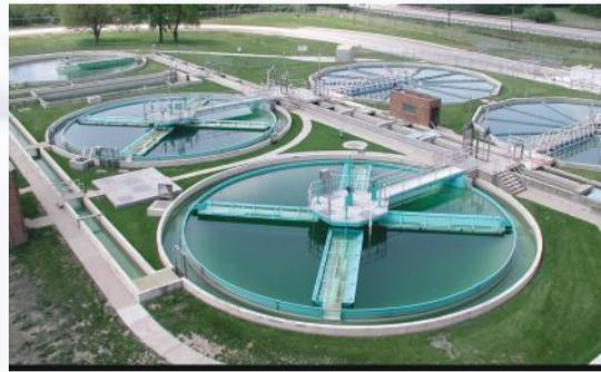
*Between 1999 and 2002, two of the original Spaulding Upflow Clarifiers were converted to larger, state-of-the-art helical flow Claricone units (foreground).*
