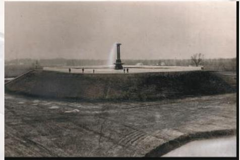
*Water pumped from the Sangamon River was temporarily stored in this reservoir before being distributed to customers.*
