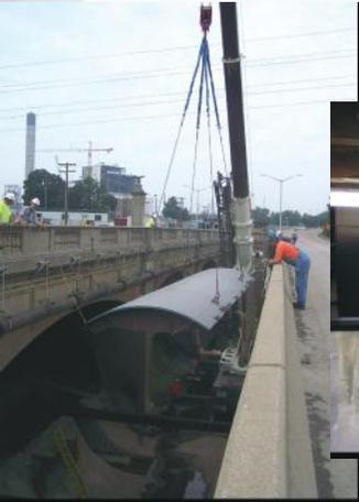
*The replacement drum for the Spaulding Dam gate number two is lowered into position (November 2008).*
